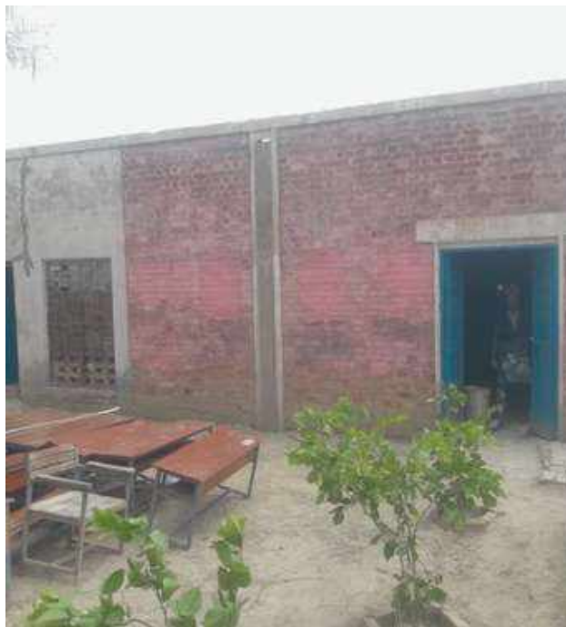
One of schools before intervention
