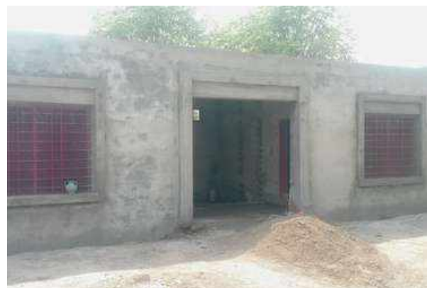
A two room house under construction
