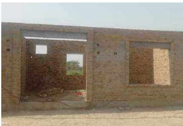
A one room house under construction
